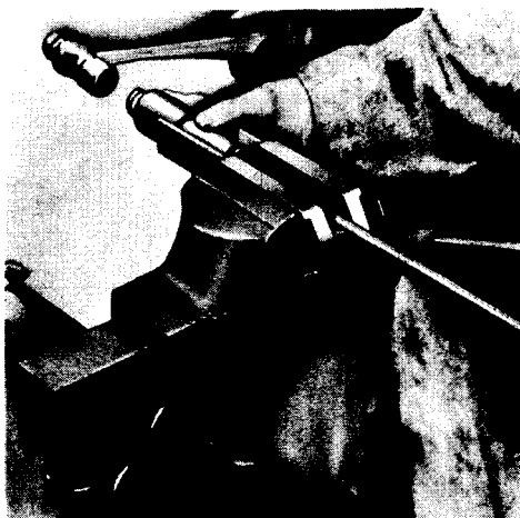
Figure 110 — Flaring Brake Tube
