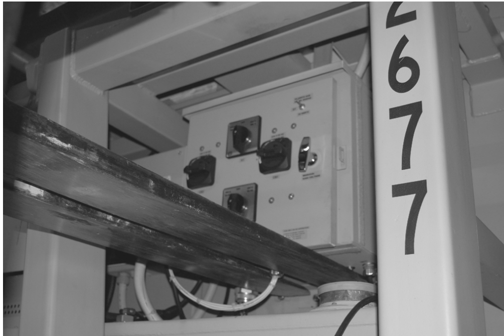
Figure 23. Lifting Power Box with Forklift.
