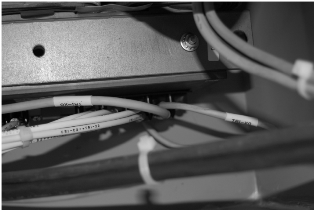
Figure 17. Removing TR1-X0 Wires from X0 Terminal.
