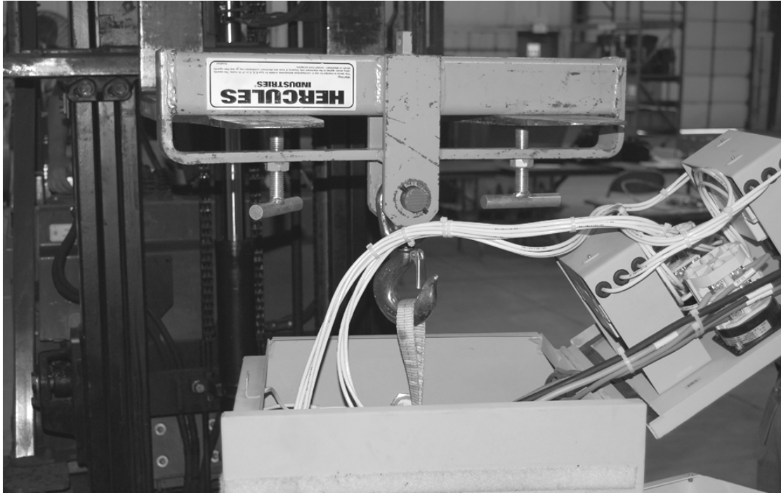
Figure 20. Lifting Transformer from Power Box.
