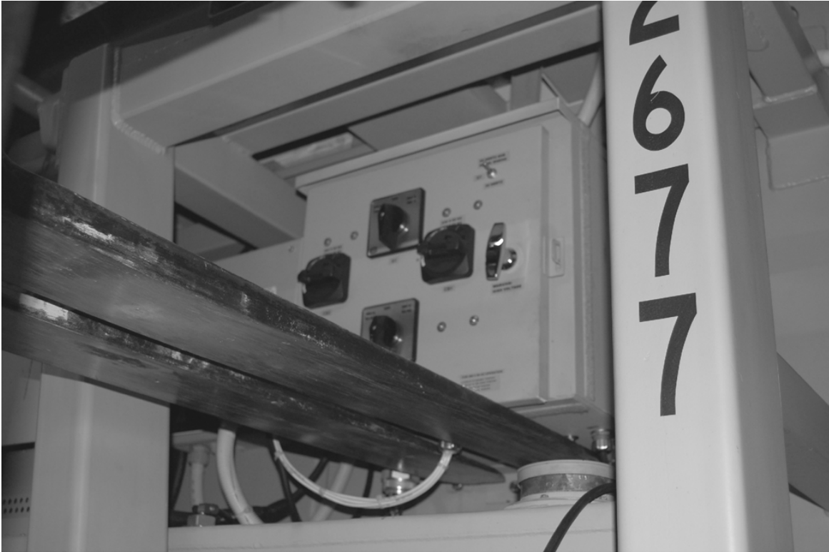
Figure 10. Positioning Forklift Entering Power Box.
