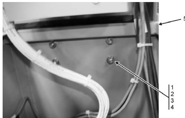
Figure 15. Electrical Box Removal.
