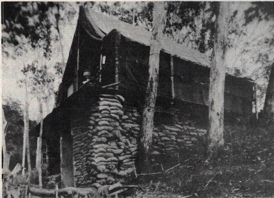
THE SEMI-DUGOUT ARRANGEMENT OF A NEW GUINEA SHIP-TO-SHORE RADIO STATION SIMPLIFIES THE PROBLEM OF PROTECTION.
