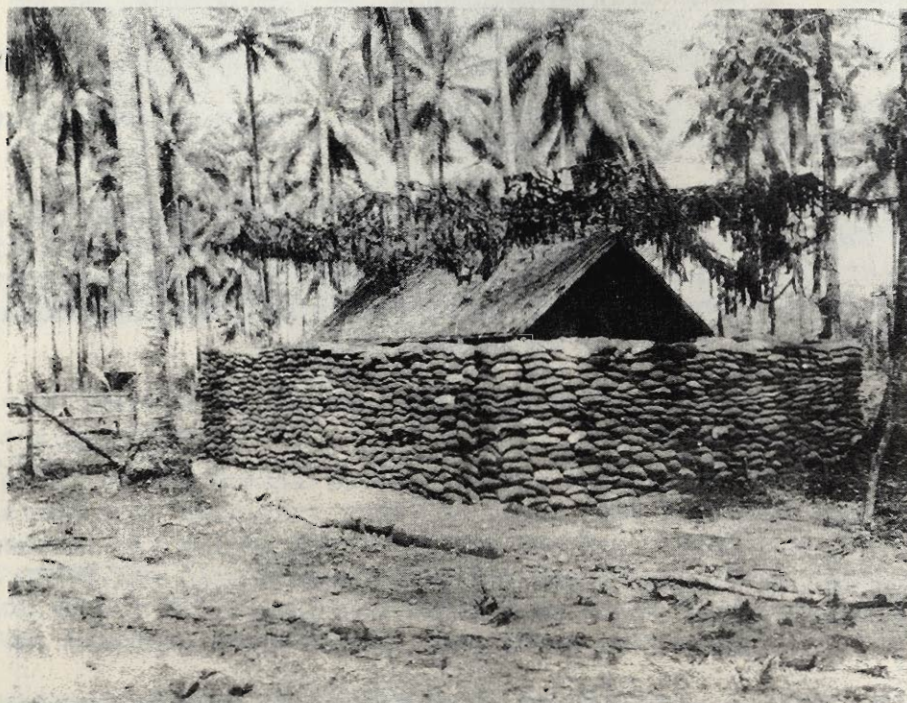
A TRANSMITTER SHACK WITH ITS CAMOUFLAGE NET OVERHEAD AND SANDBAG PROTECTION AGAINST SNIPERS AND SHRAPNEL.
