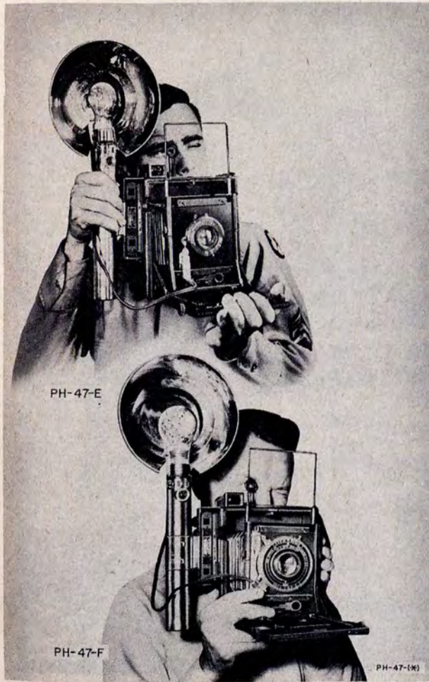
Figure 13. Cameras PH-47-E and PH-47-F.
