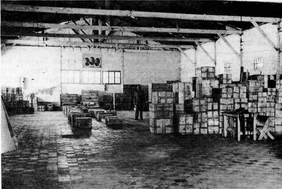
A STORAGE DEPOT KEEPS SUPPLIES SEGREGATED AND UNDER COVER
