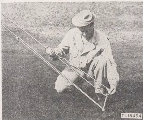
Figure 14. Looping hoist rope over stake.
