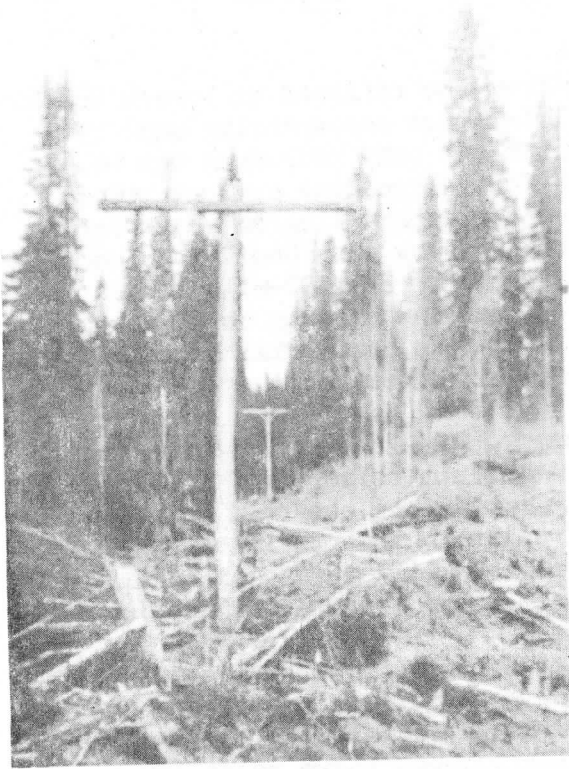
SEPARATE RIGHT-OF-WAY IS CLEARED FOR THE LINE WHERE DISTANCE CAN BE SHORTENED.
