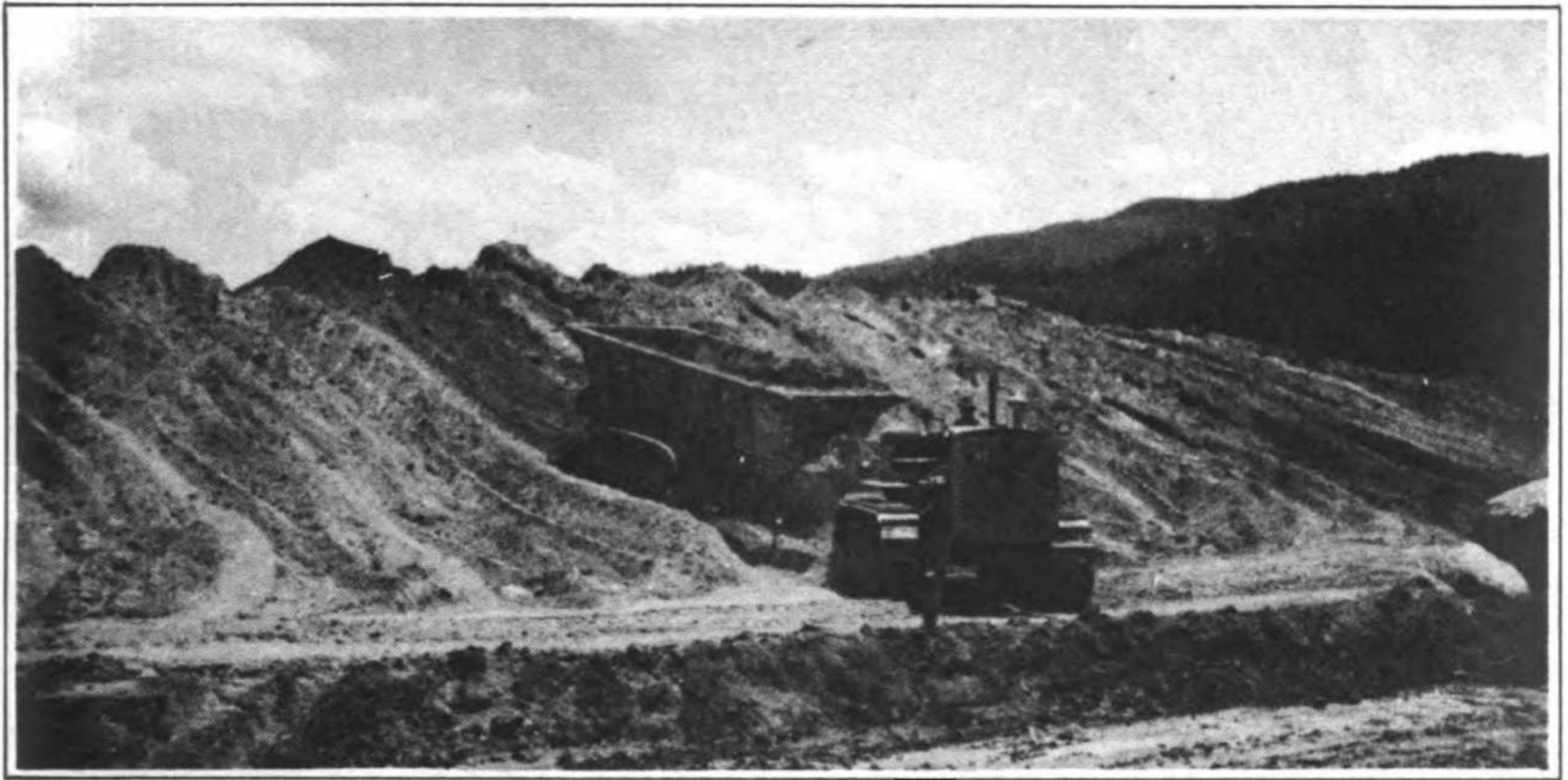
DISCHARGING MATERIAL OVER END OF FILL Fig. 4
