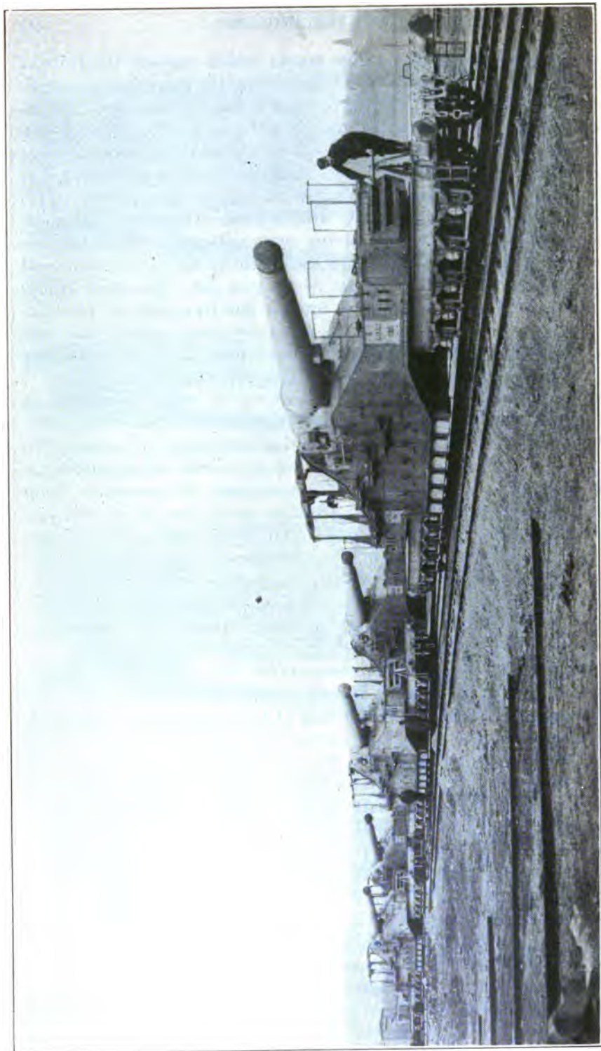
FIG. 34.—306-mm. railway mount (Schneider) for U. S. 10-inch guns, models 1888 and 1895.
