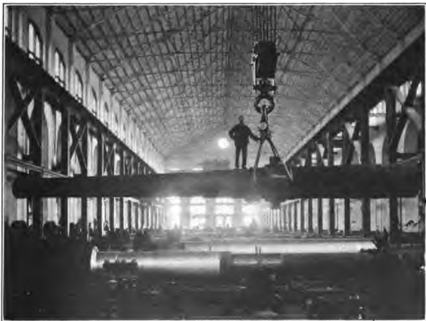
FIG. 208.—Gun shop Watervliet Arsenal with 14-inch gun suspended from travelling crane.
