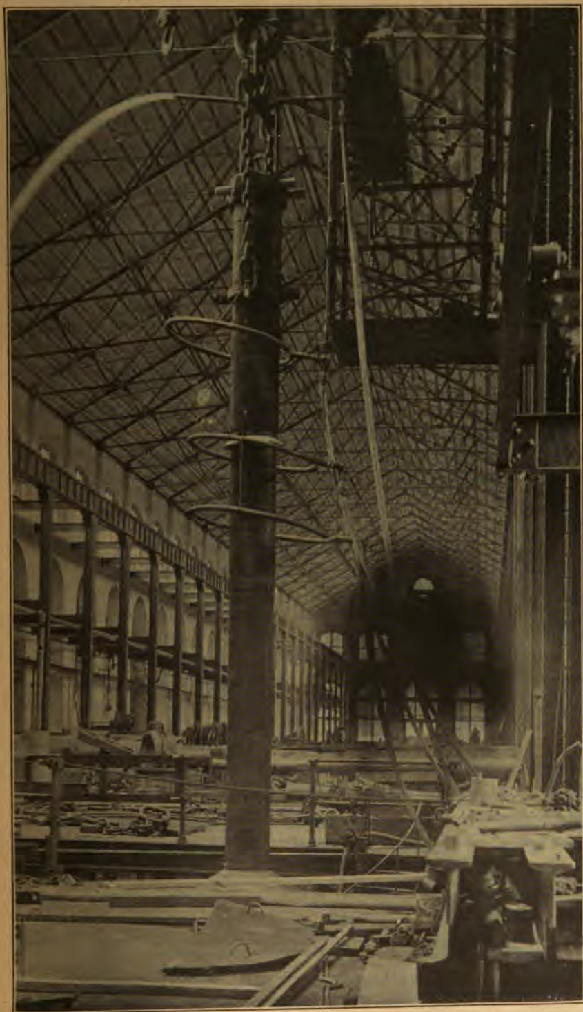
FIG. 5.—Equipment for cooling tubes at shrink pit, Watervliet Arsenal. Shrinking of 14-inch wire-wound gun.
