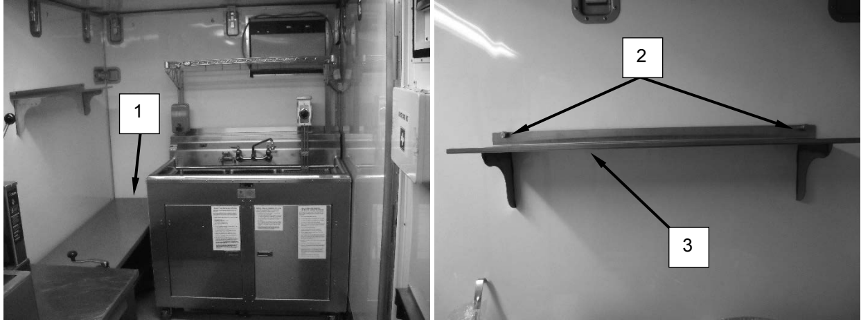
Figure 22. Install Utility Table and Spice Rack.
