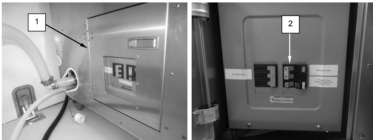
Figure 3. Resetting the Immersion Heater Circuit Breaker.
