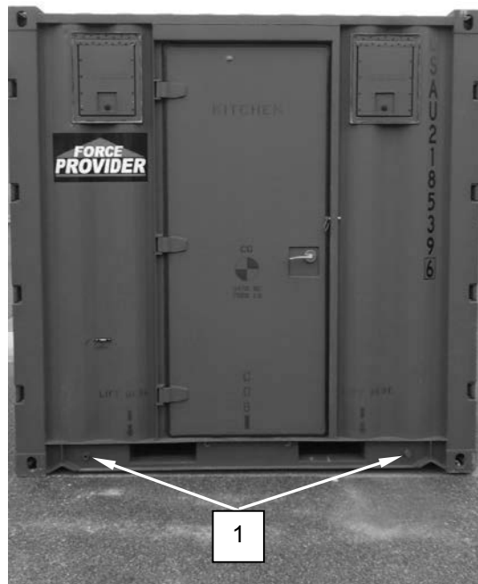
Figure 1. Remove Drain Plug.
