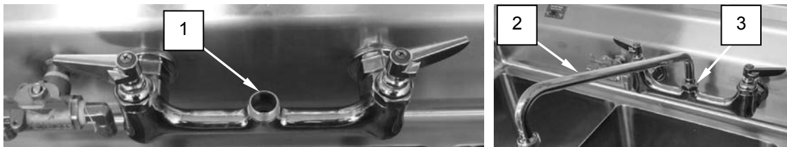
Figure 17. Install Gooseneck.
