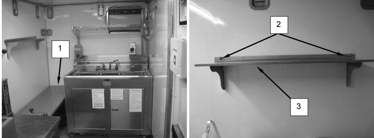
Figure 11. Install Utility Table and Spice Rack.
