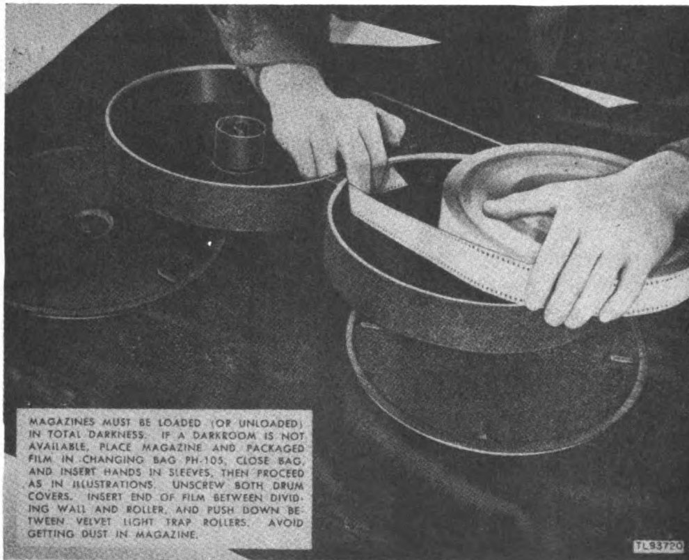
Figure 13. Loading magazine: threading film through light trap.
