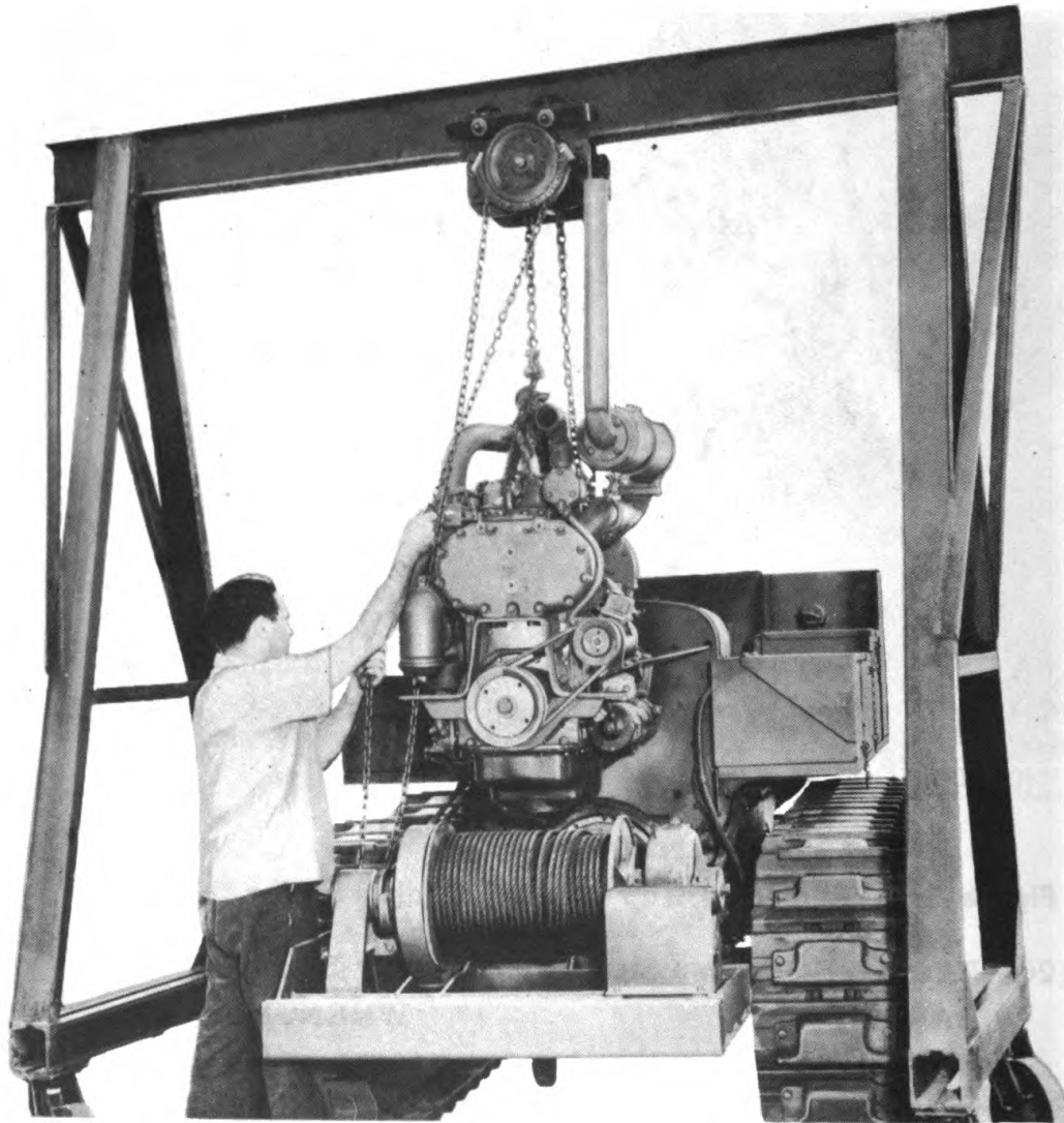
Figure 20 — Removing Engine from Tractor
