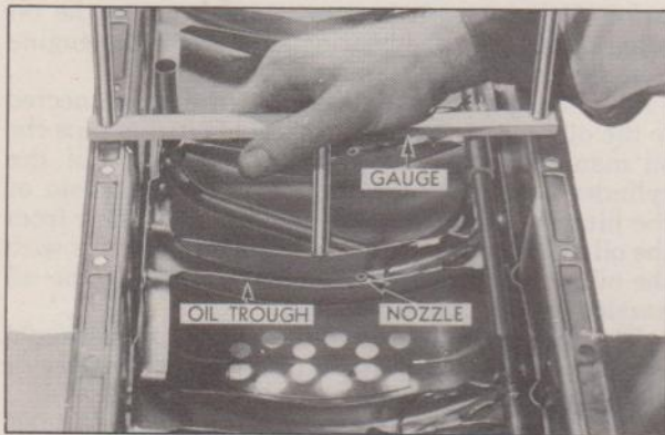
Fig. 37—Checking Oil Trough Depth
