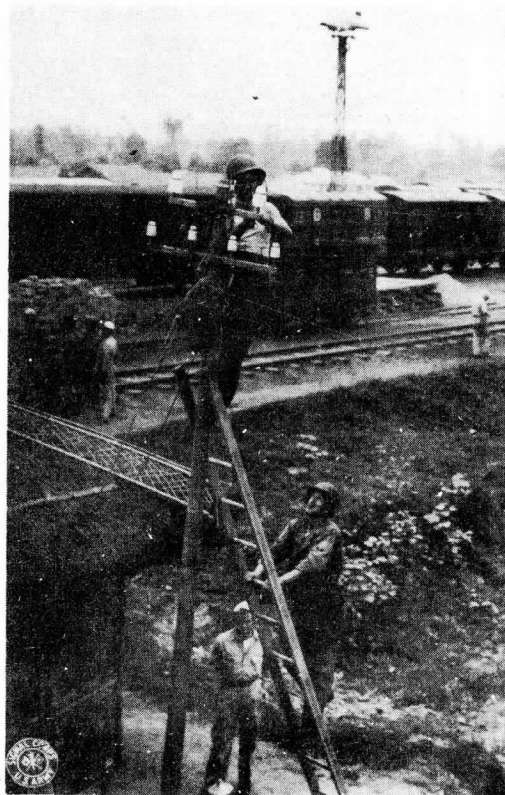
OVERHEAD LINES PARALLEL RAILROAD
