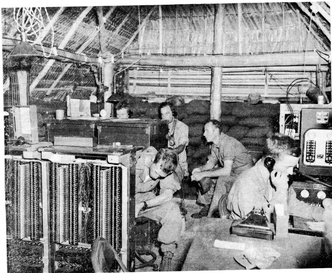
A THATCHED ROOF AND SANDBAG WALLS PROTECT THIS JUNGLE TELEPHONE EXCHANGE.
