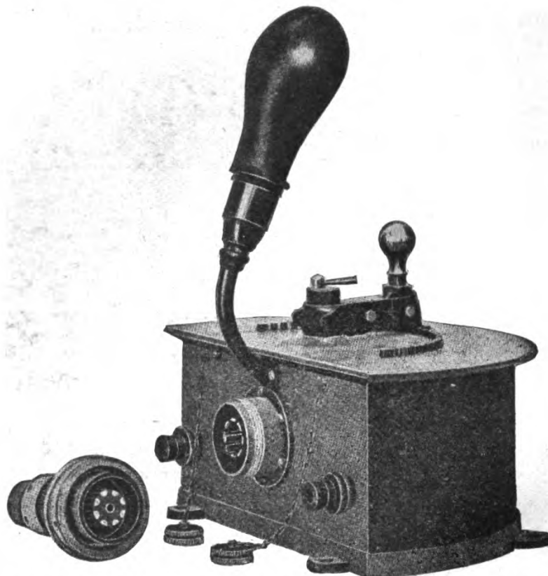
FIG. 35.—Ardois system keyboard, showing receptacles for cables.
