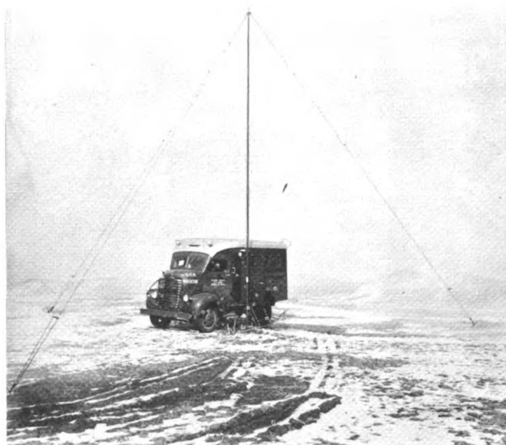
FIG. 6 TRUCK, EXTERNAL VIEW SHOWING ERECTED ANTENNA
