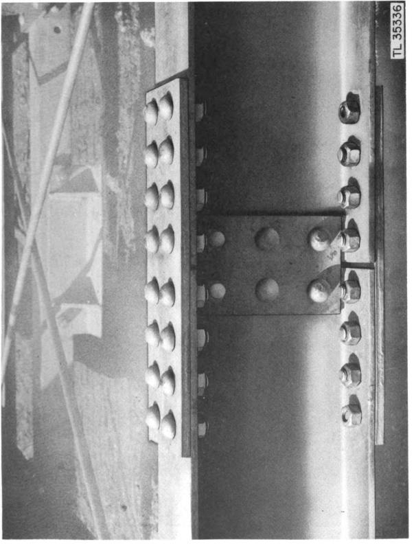
Figure 3. Junction of main beams.
