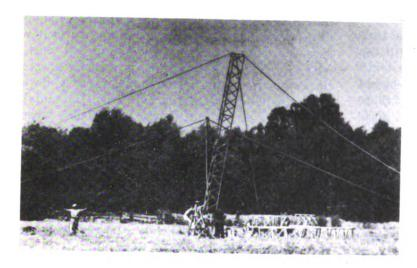
Figure 23. Tower erection, first phase.
