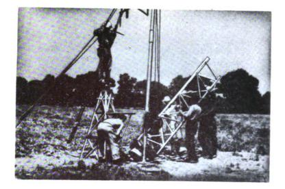
Raising tower section into vertical position so that it can be raised for connection to upper part of tower.
