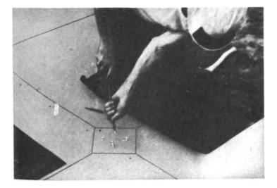
Placing interior floor panel. The rabbets, screeds and splines have been carefully cleaned of earth or gravel before the panel is shoved into place.
