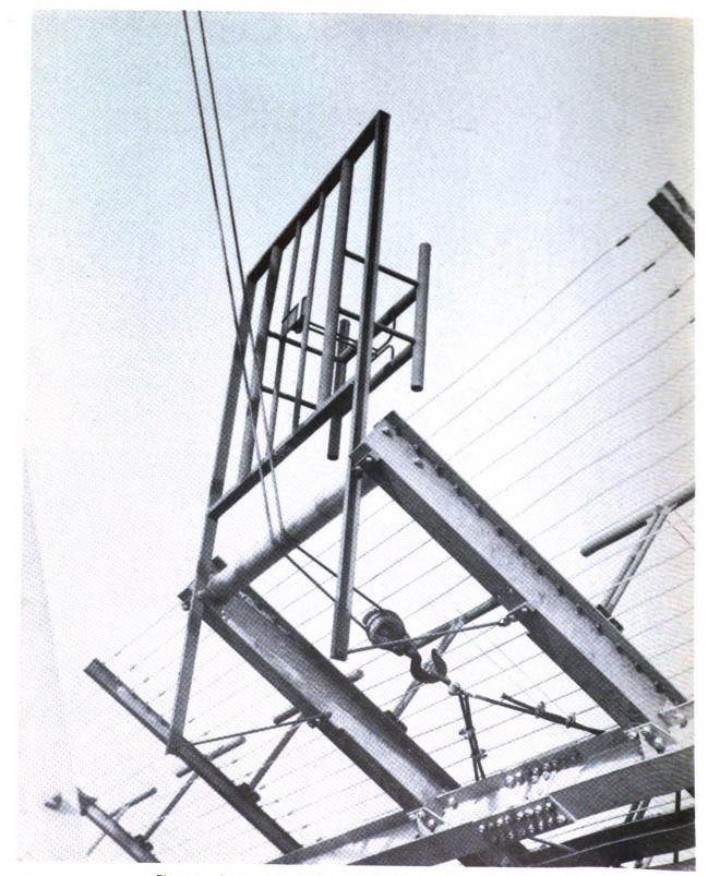
Figure 9. Antenna AN-161, IFF installation, hoisting sling attached, rear view
