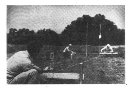
Placing batter boards and establishing building line. Note the stanchion bars placed upright which are used as sight guides for establishing tower locations and building lines.
