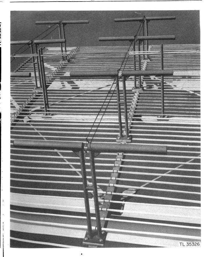
Figure 15. Antenna AN-161, vertical transmission line connections.
