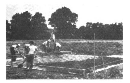
Covering waterproofing. A thin layer of earth has been spread on waterproofing to permit foot traffic and placement of wood screeds.
