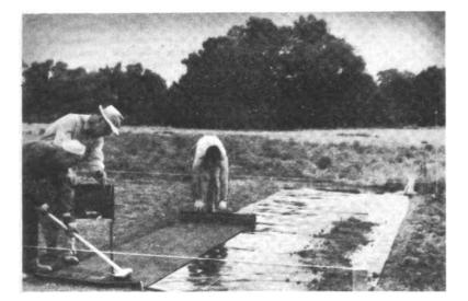
Placing waterproofing after earth has been leveled and tamped. Note that felt is unrolled into place on top of adhesive.
