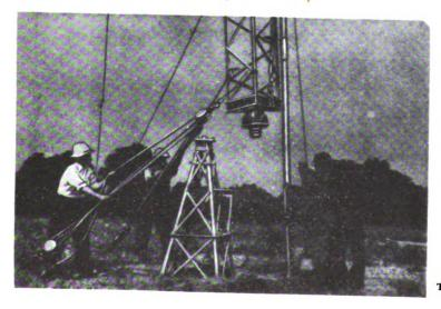
Swinging tower onto base. The kick anchors play an important part in this operation.
