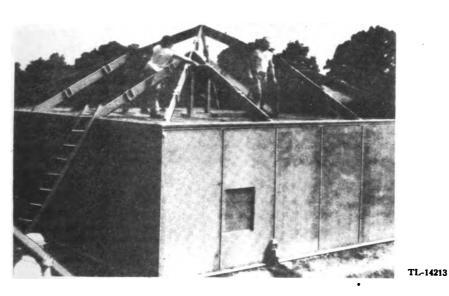
Figure 13. Placing wall panel, ceiling panel, and roof rafters.
