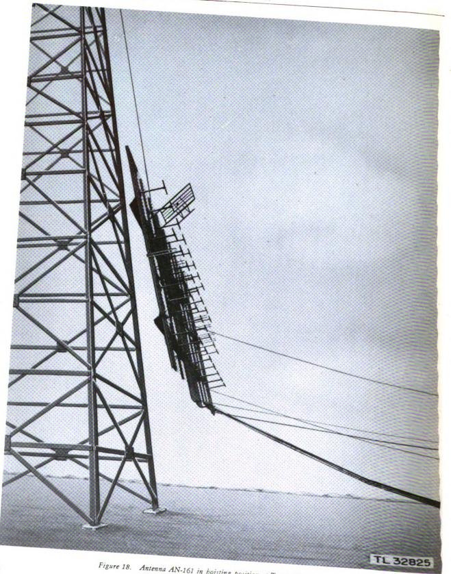
Figure 18. Antenna AN-161 in hoisting position at Tower TR-20A
