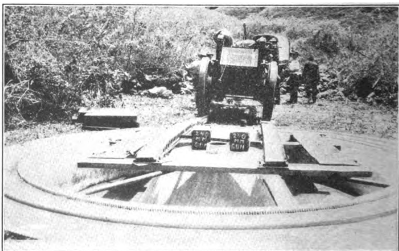
FIGURE 86.—360° emplacement with top carriage in position for mounting. Jack foot blocks in position
