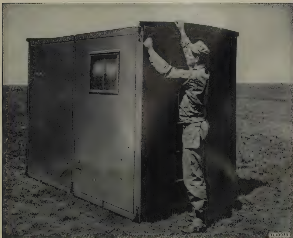
Figure 46. Shelter HO-20-B, tightening wingbolts.
