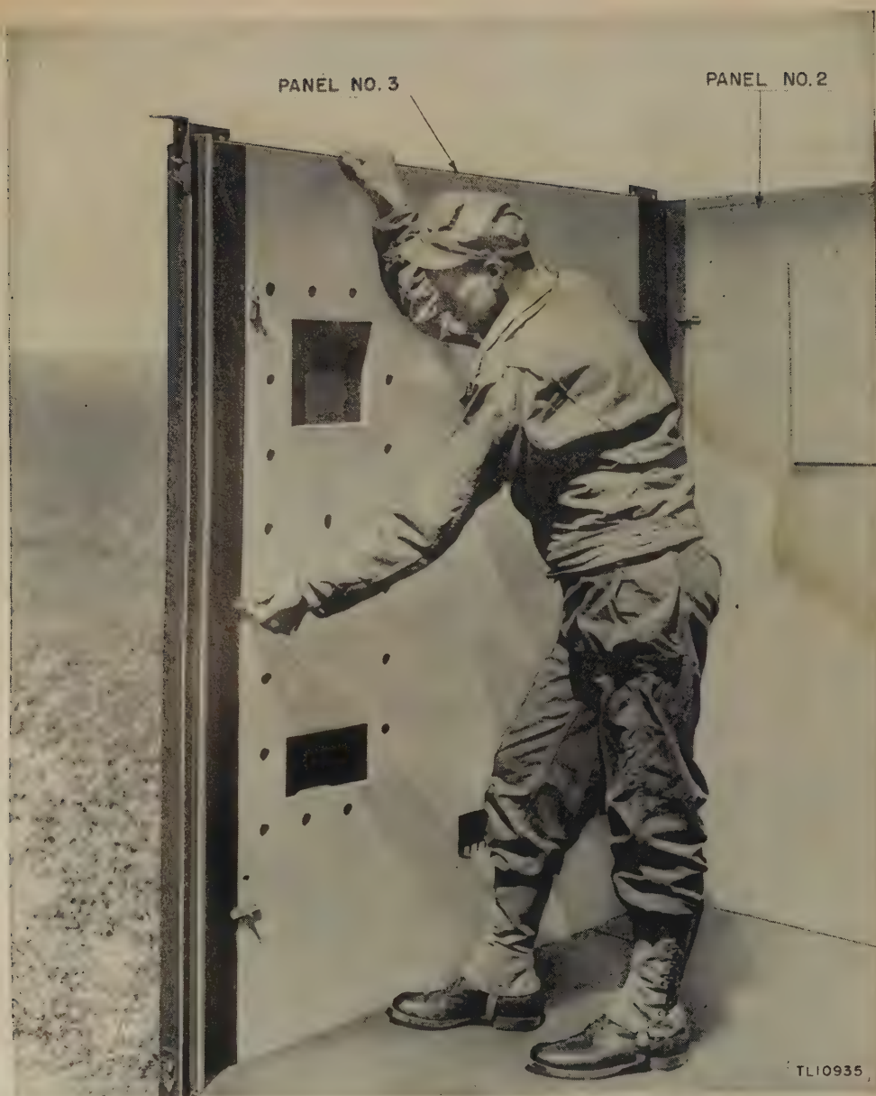
Figure 44. Shelter HO-20-B, fastening panel.
