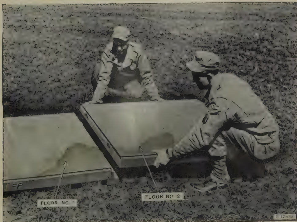
Figure 40. Shelter HO-20-B, floor assembly,
