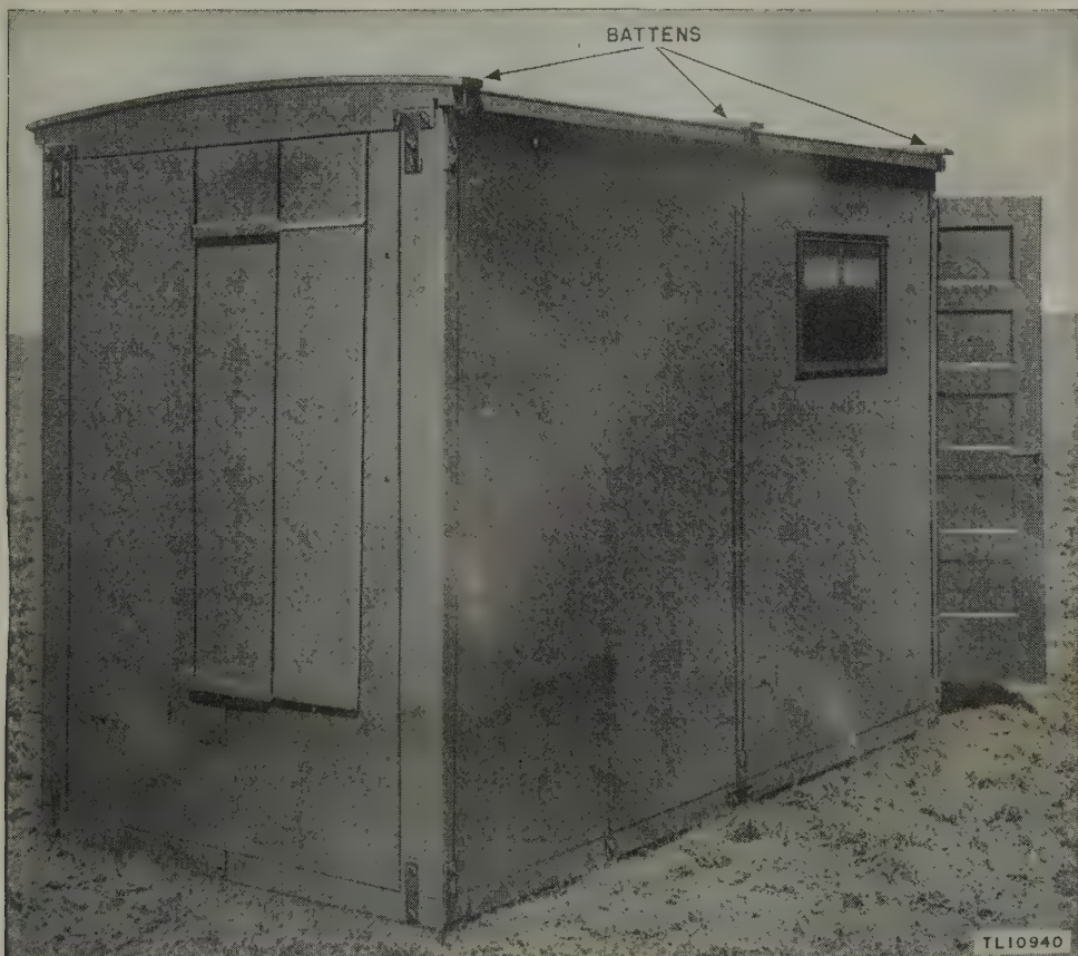
Figure 48. Shelter HO-20-B, battens fastened over roof.
