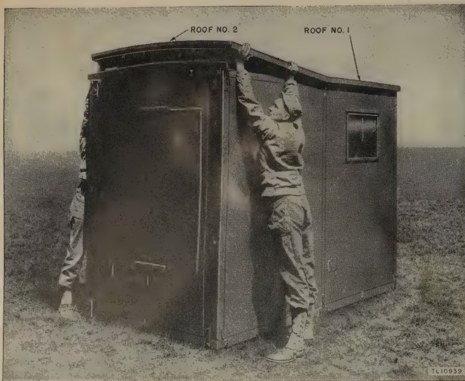
Figure 47. Shelter HO-20-B, installing roof sections.
