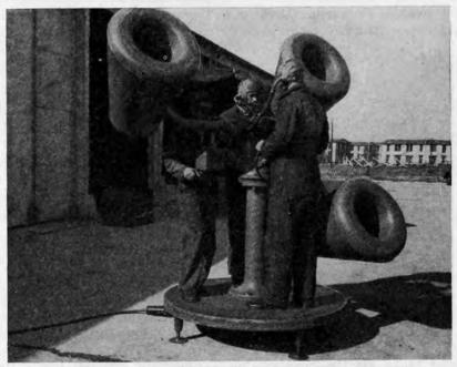
FIGURE 133 .- Sound locator, M2, in listening position.
