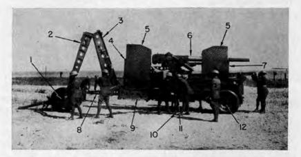
FIGURE 166.—Emplacing 3-inch AA mount, M2 (front bogie removed, front outriggers being placed and jacks manned).
