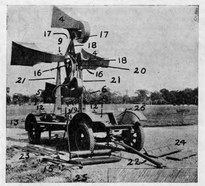
FIGURE 131 .- Sound locator, M1A1, in listening position.
