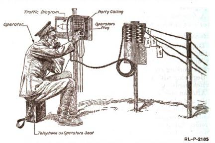
Fig. 10.—Operator answering a call on the monocord switchboard.
