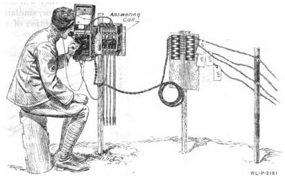
Fig. 14.—Operator answering a call with the monocord switchboard operator's set.
